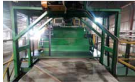
After material spillage improvements at forming station
